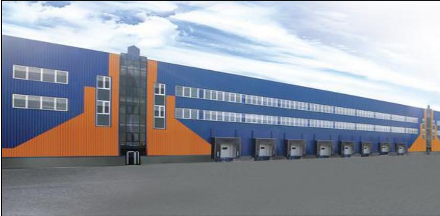
The building is divided into six independent sections (each at least 6,400 sq m), with internal clear ceiling of 12m height and industrial flooring constructed with anti – dust overlay quartz finish. The terminal accommodates 90 parking spaces for cars and trucks, as well as 24 hour security and municipal provided sewage, water and garbage collection.
